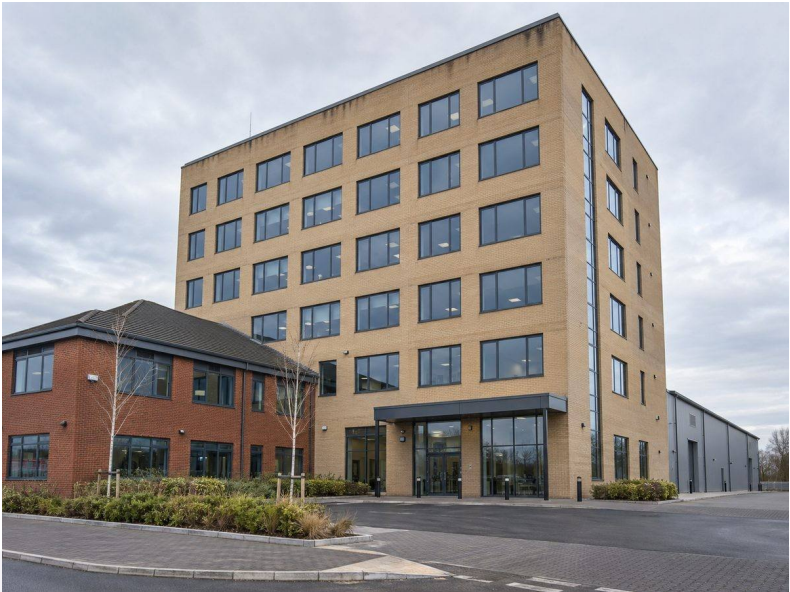
Photo 1: Main office block and office wing, front
