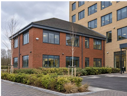
Photo 16: Office wing, front
