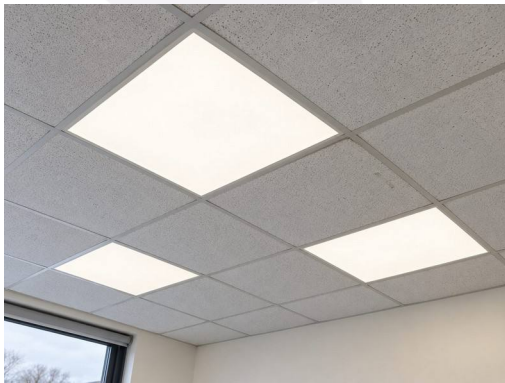
Photo 11: LED panels, typical office floor
