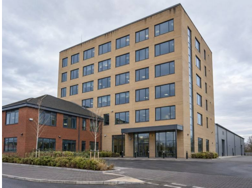
Photo 1: Main office block and office wing, front
